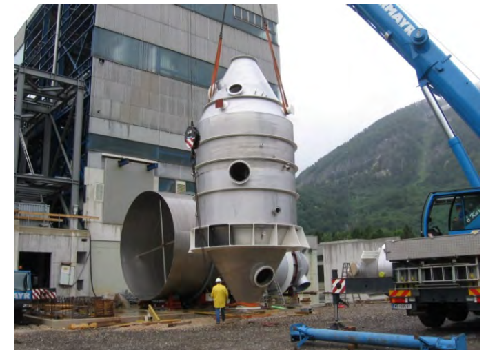
Site fabrication and mounting (Austria) Evaporation crystallizer \varnothing 6.400 mm, overall length 18.700 mm, 56 t, 1.4562
