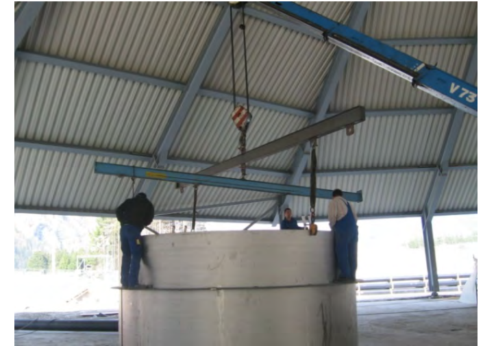
Site fabrication and mounting (Austria) Evaporation crystallizer \varnothing 6.400 mm, overall length 18.700 mm, 56 t, 1.4562
