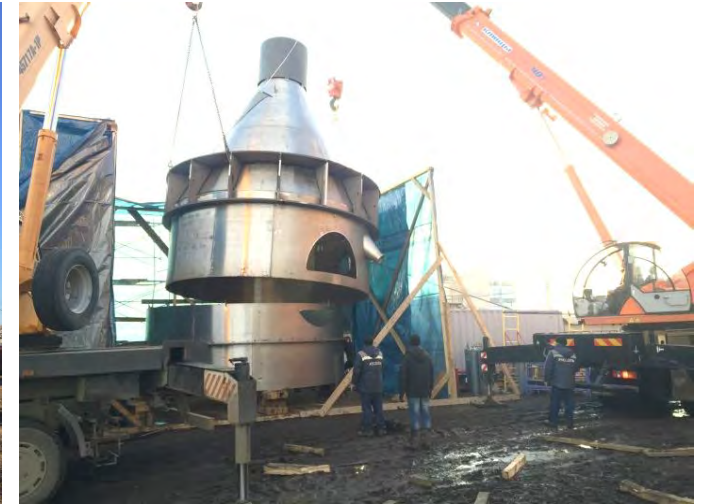
Site fabrication and mounting (Russia) Evaporating crystallizer Ø 5.400 mm, overall length 21.800 mm, 40 t, 1.4562
