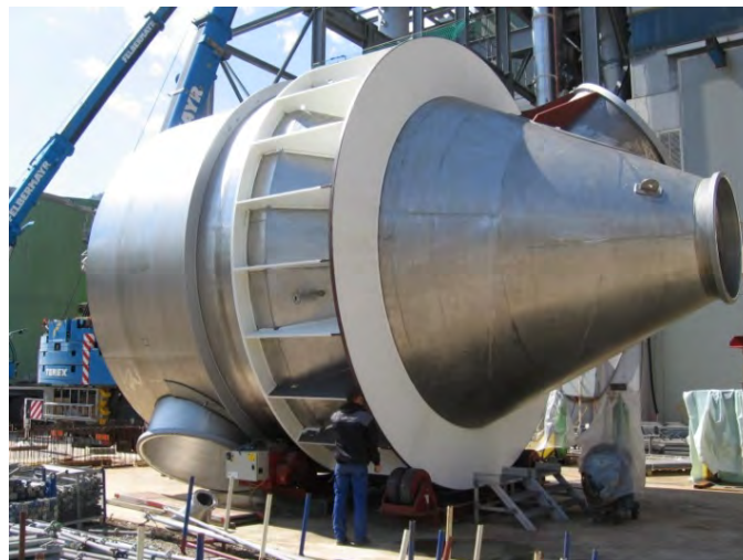
Site fabrication and mounting (Austria) Evaporation crystallizer \varnothing 6.400 mm, overall length 18.700 mm, 56 t, 1.4562
