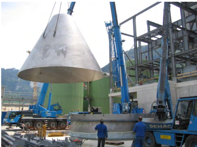
Site fabrication and mounting (Austria) Evaporation crystallizer \varnothing 6.400 mm, overall length 18.700 mm, 56 t, 1.4562
